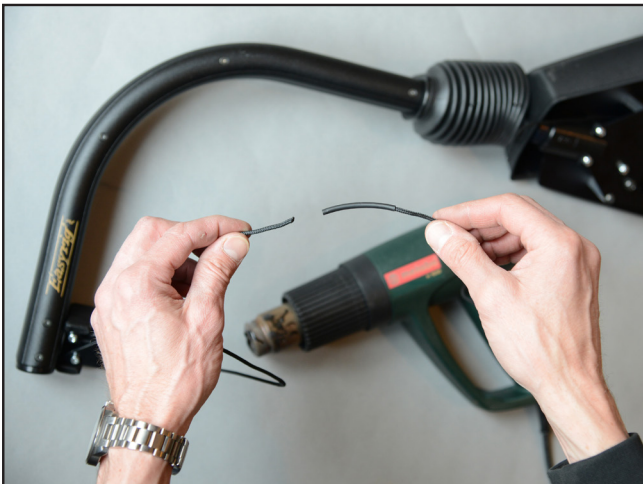
3. Mount shrink tubing on the two line ends.
